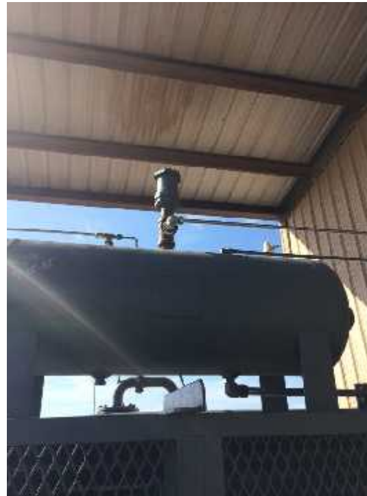
Coolant tank vented via tubing line and ball valve
