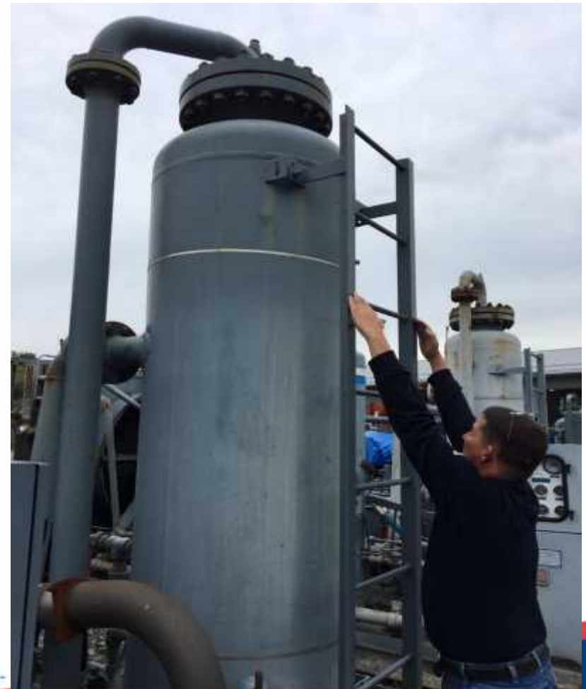
Fixed ladder instead of a work surface
