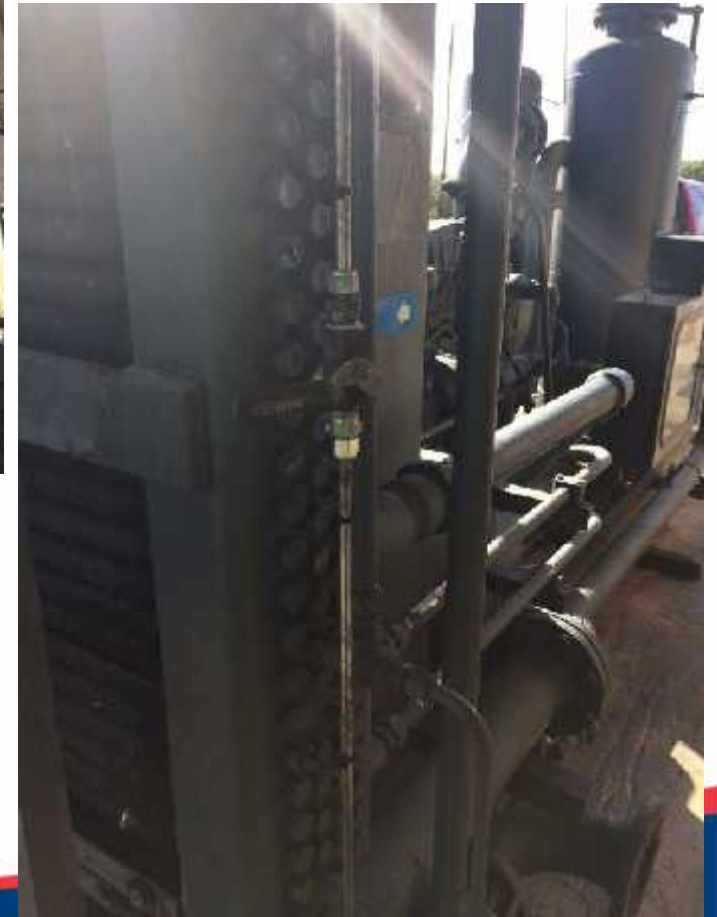
Coolant tank vented via tubing line and ball valve
